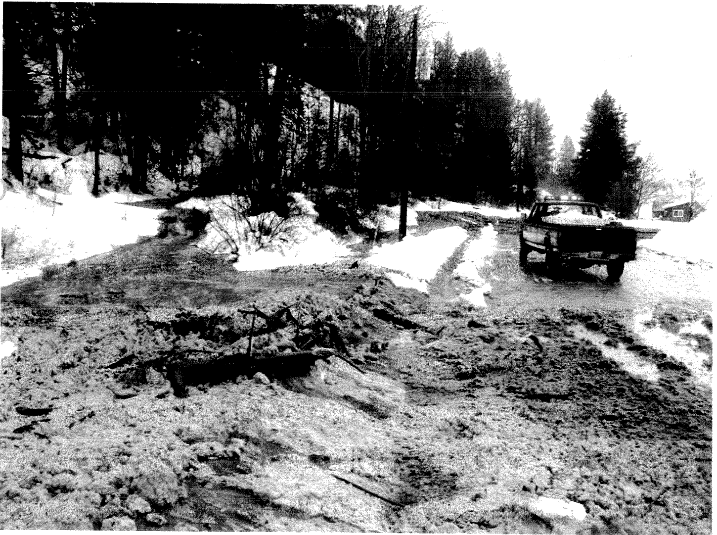
A second slide on Red Bridge Road.
